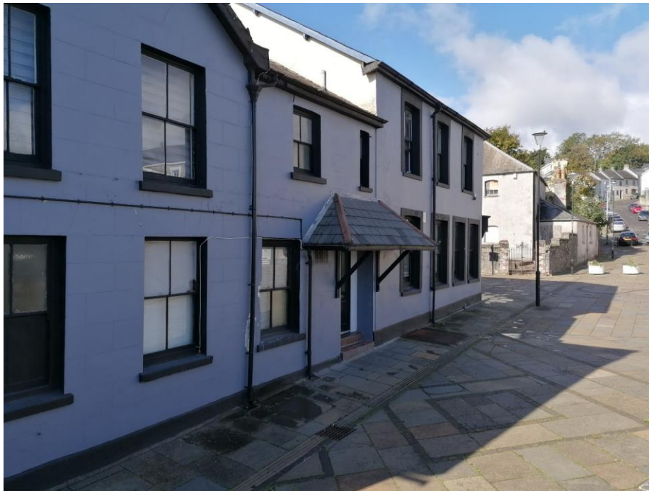
Photograph of site's front elevation
